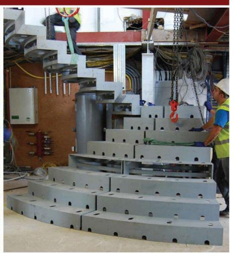
The stairs' steel structure consists of continuous steel folded plates braced between a zig-zag stringer profile to create a mono-coque structure to be fully clad. At it's widest point the stair is a grand 3.5 meters, tapering down to 1 meter.
